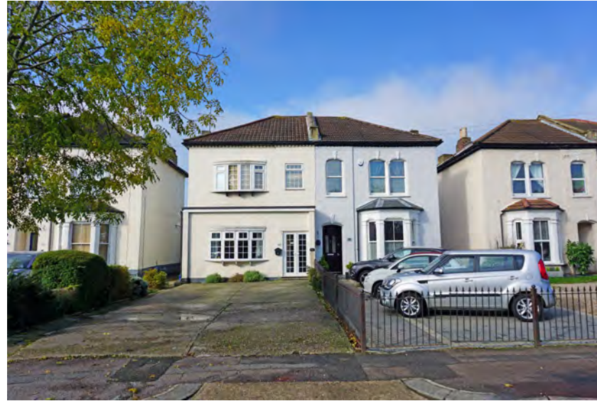
Inappropriate boxy modern extension to the ground floor and bow window to first floor which replace the original bay and sash windows. There are opportunities to enhance this building through the reversal of inappropriate changes
