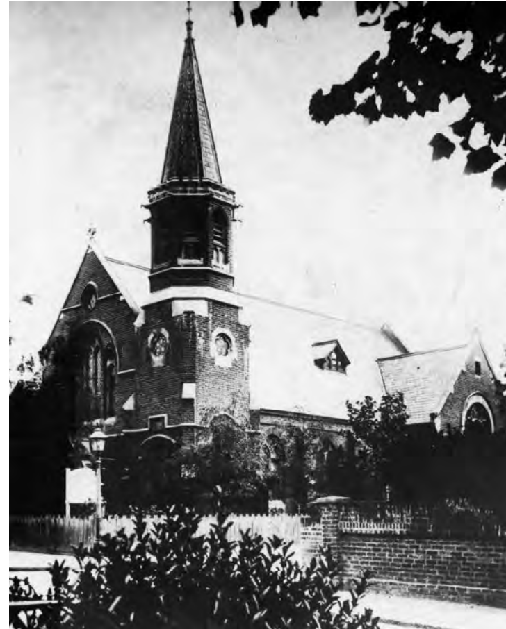
St Georges Presebytarian Church now demolished
