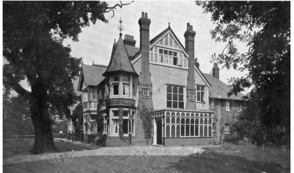
The grand façade of Barons Court as seen from Avenue Road. The decorative turret and side porch would have been very noticeable in the streetscene. The already mature trees of 'Mill Lane' can be seen in front of the building.
