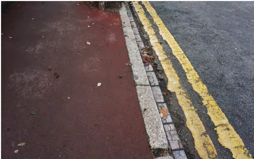
Red asphalt pavement, glazed brick drainage channel and granite kerb
