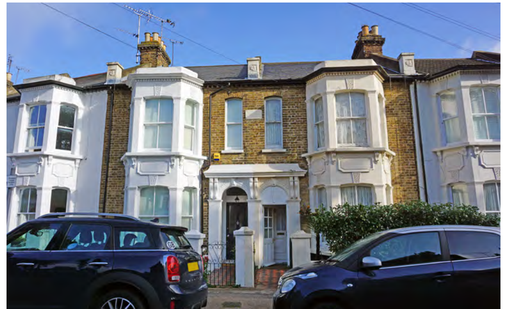
Late Victorian terraces dating to 1874 along Avenue Road
