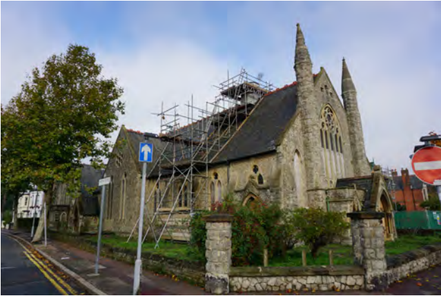
Park Road Methodist Church, currently vacant
