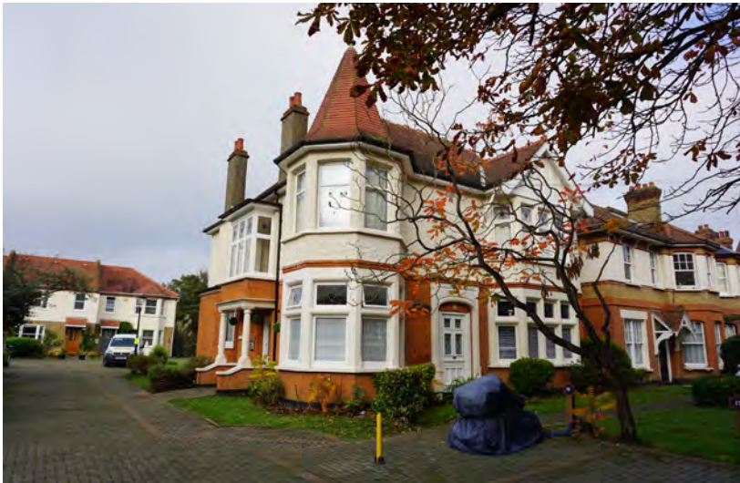
Architectural detailing focuses on strong vertical emphasis across the Conservation Area
