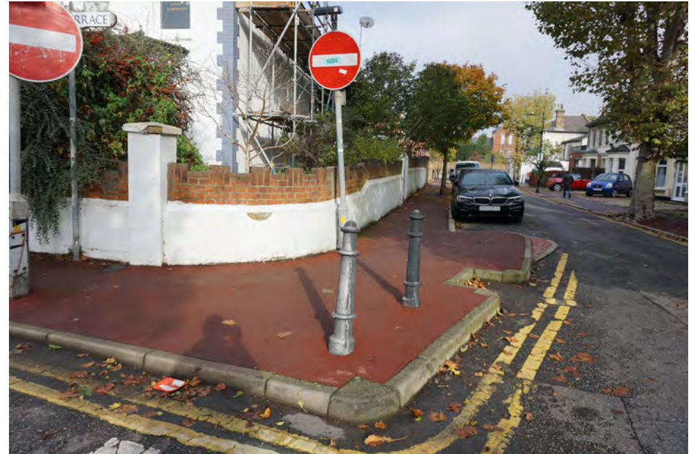
Good quality red tarmac pavement but multiple signs and bollards, along with wide yellow lines
